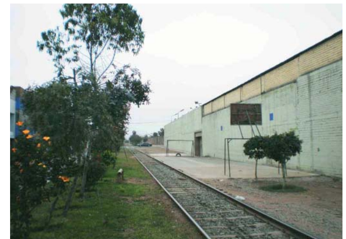
Facilities on Enrique Meiggs Street.
